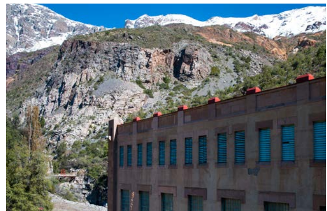
Queltehues Hydroelectric Power Plant in San José de Maipo
