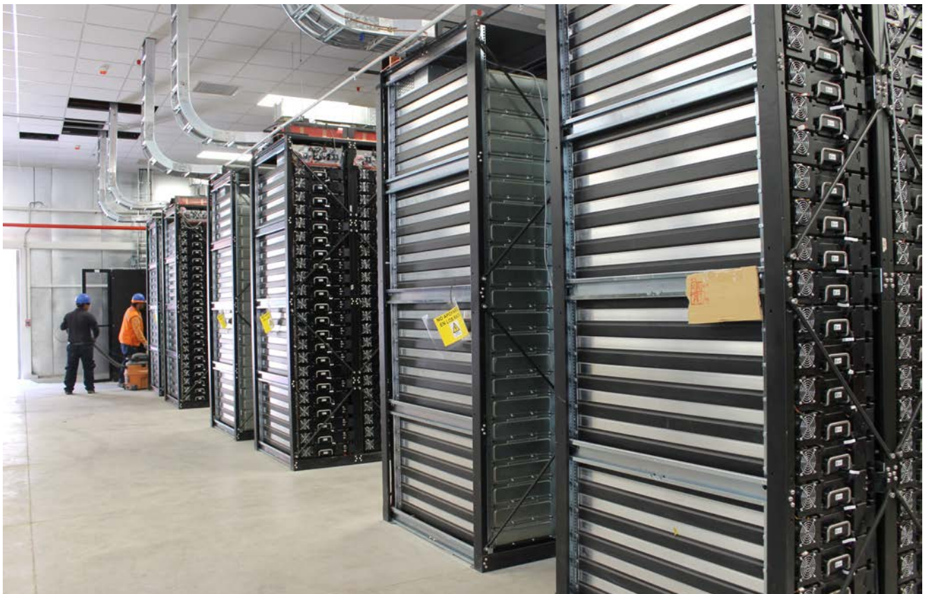
Virtual Reservoir, the world's first energy storage system, integrated into a run-of-the-river hydroelectric power plant.
